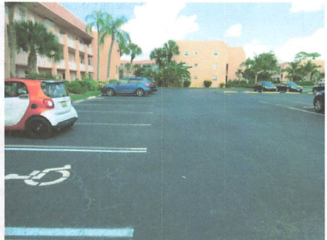
PARKING AND PAVEMENT
