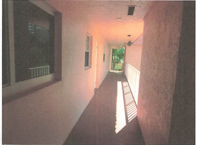
VIEW OF ELEVATED WALKWAY
