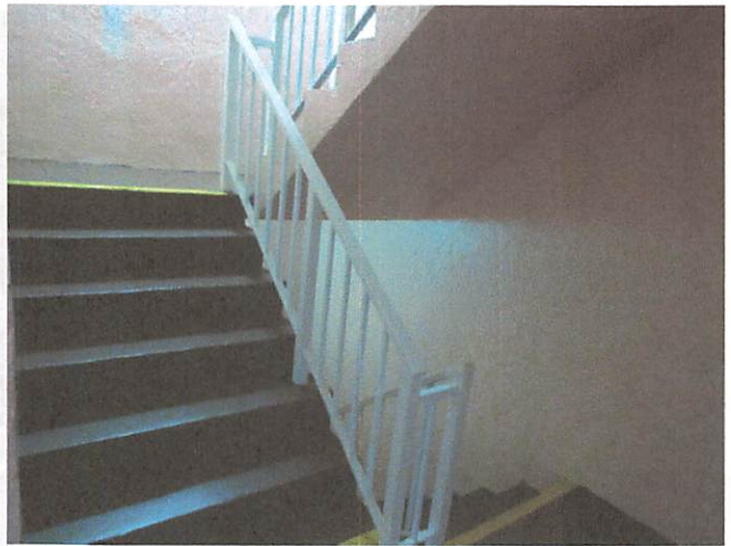
VIEW OF EXTERIOR STAIRS
